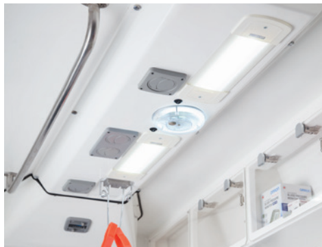
Cabin ceiling services panel
